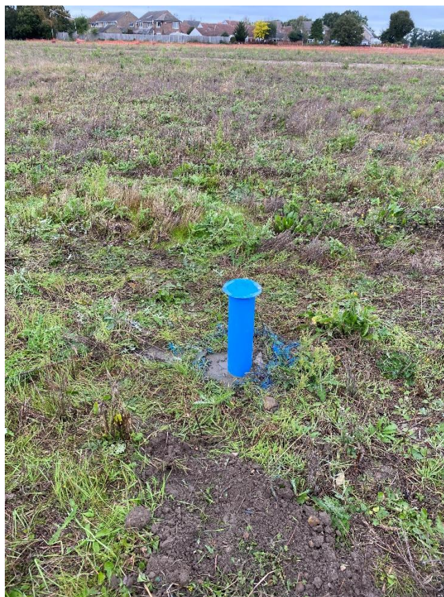
Photograph 14 – Installation cover. Subject: WS403
